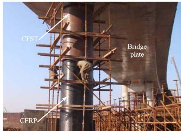
Figure 2. An Engineering Practice of C-CF-CFRP-ST Columns Used in Nanjing City, Jiangsu Province, P. R. China
