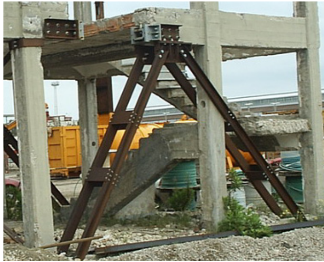
Figure 23. The Retaining Steel Structure
