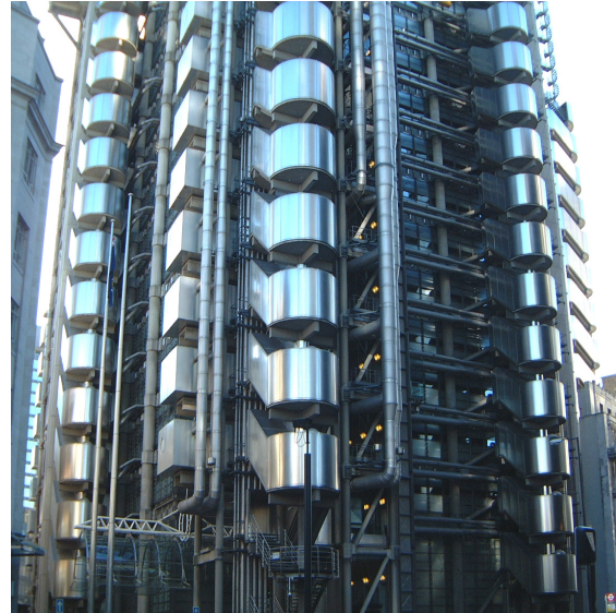
Figure 3. Services and Stairs Located on the Exterior of the Lloyds Building in London
