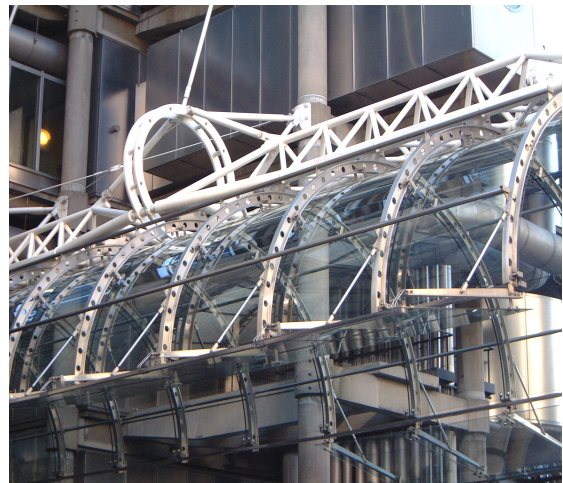
Figure 5. Stainless Steel Entrance Canopy of Lloyds Building, London
