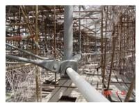
Figure 5. Sliding Cable-strut Joint
