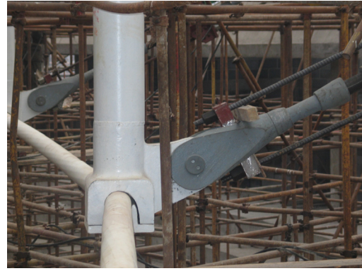
Figure 8. Sliding Cable-strut Joint
