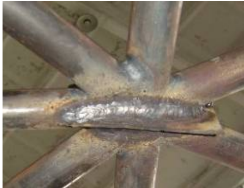
Figure 7. Node in Single-layer Latticed Shell
