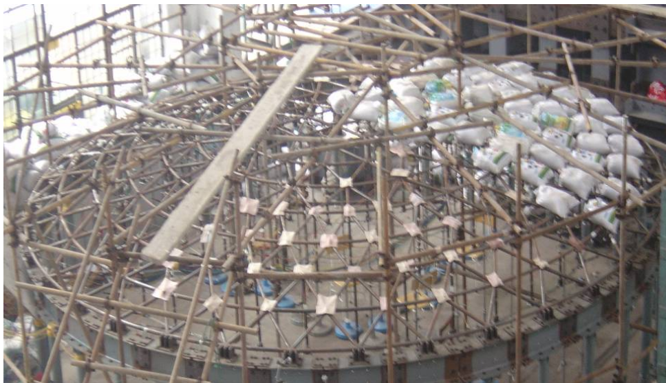
Figure 13. Loading of Heap Load
