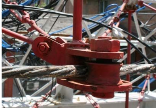
Figure 4. Real Photo of the Sliding Cable-strut Joint
