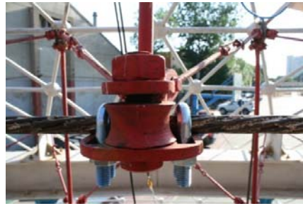
Figure 20. U-shaped Locks to avoid Cable Sliding through the Joint
