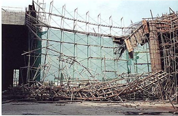
Figure 2. Collapse Scene of Single-row Steel Scaffolds Underneath the Beam of the Entrance Lobby of Chayi Tzu-Chi Hospital during Construction in Chayi County, Taiwan
