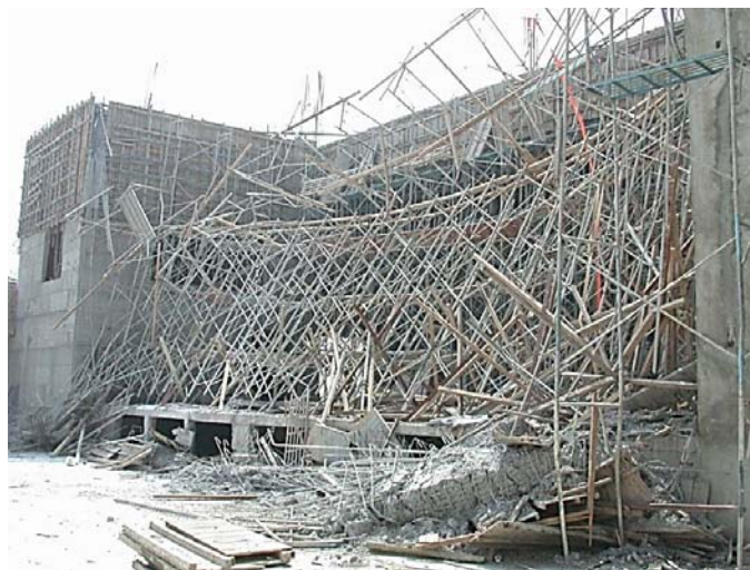
Figure 4. Collapse Scene of Single-row Steel Scaffolds Underneath the Beam of the Auditorium of Mingdao College of Management during Construction in Zhanghua County, Taiwan
