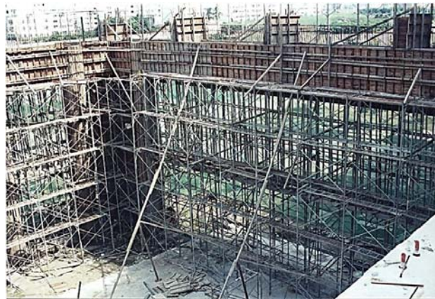
Figure 1. Setup of Single-row Steel Scaffolds Underneath the Beam of the Entrance Lobby of a Hospital during Construction
