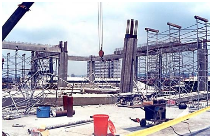
Figure 3. Collapse Scene of Single-row Steel Scaffolds of RT-mart Mall under Semi-prefabrication Construction in Zhanghua County, Taiwan
