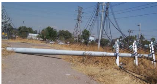
a) Power pole collapse. Electrical substation, Mexico City, January, 2009
