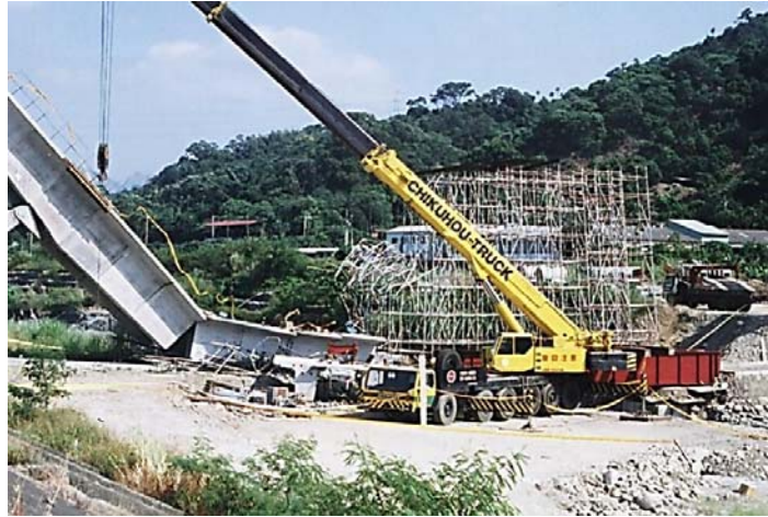
Figure 1. Collapse of Falsework in Construction of Access Bridge of 921 Earthquake Museum in Taichung, Taiwan
