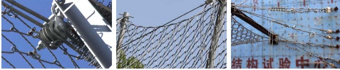
(a) Connection between support rope and steel post
