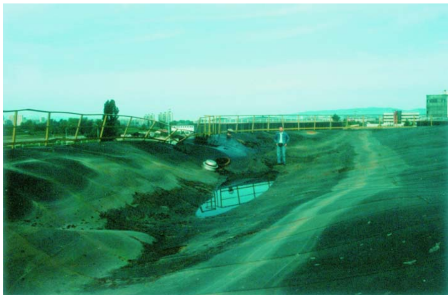
Figure 6. Form of Depression on the Roof Surface
