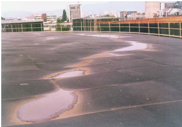
Figure 10. Depressions on the Roof Surface
