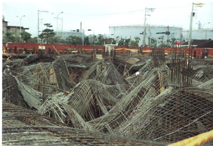
Figure 3. Collapse Scene at Construction Site of Xinzhu Chemical Engineering Warehouse Mall, Taiwan
