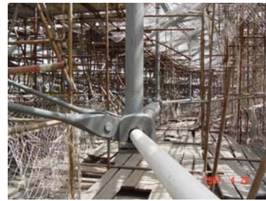
Figure 5. Sliding Cable-strut Joint
