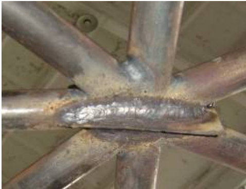
Figure 7. Node in Single-layer Latticed Shell
