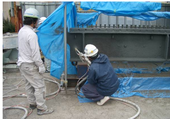
(b) Rubber-Latex Mortar Spaying Construction
