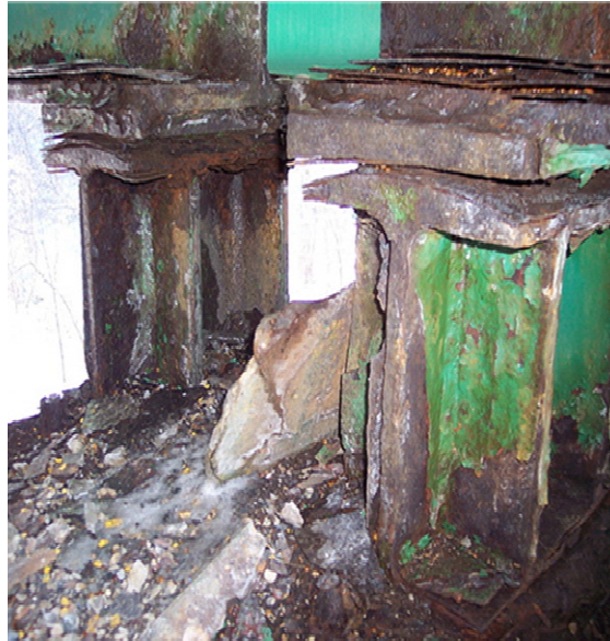
Figure 1. Corrosion Affected Elements of a Steel Bridge
