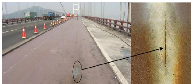
Figure 1. Cracking in Deck Plates and Along Fillet-welds Between Ribs and Deck Plates
