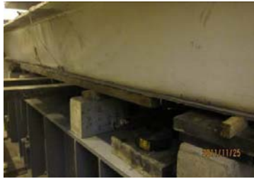
Figure 12. Strengthened by Bonding Steel Plate
