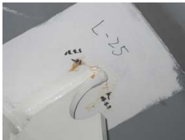
(a) Fatigue Crack at End of Vertical Stiffener
