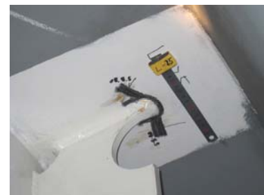
(c) ICR Treated Crack
