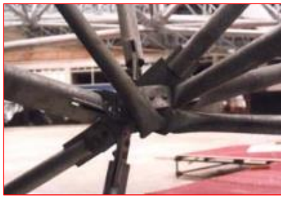
Fig. 7 Node failure [9]
