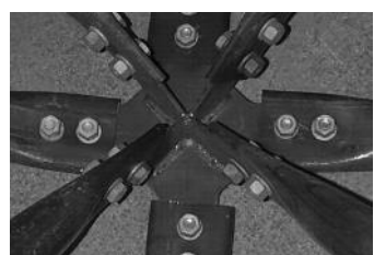
Fig. 2 Steel node [3]
