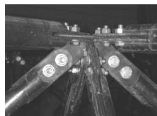
Fig. 3 Steel node made with plates [3]
