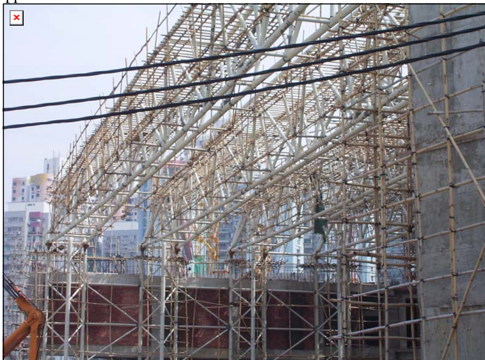
Figure 12. Stadium under construction
