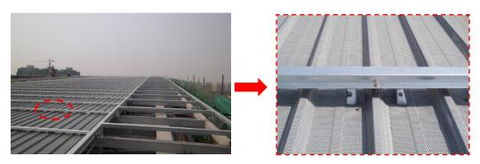
Fig. 23 Installation diagram of the base plate of metal roofing
