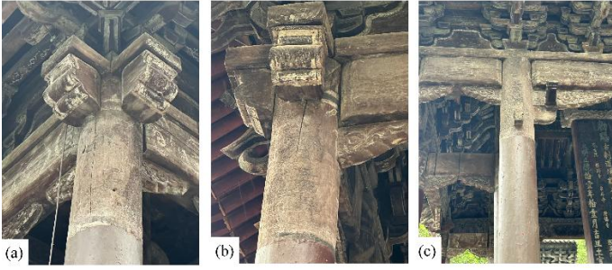
Fig. 1 Typical damage conditions of mortise-and-tenon joints in ancient timber structures
