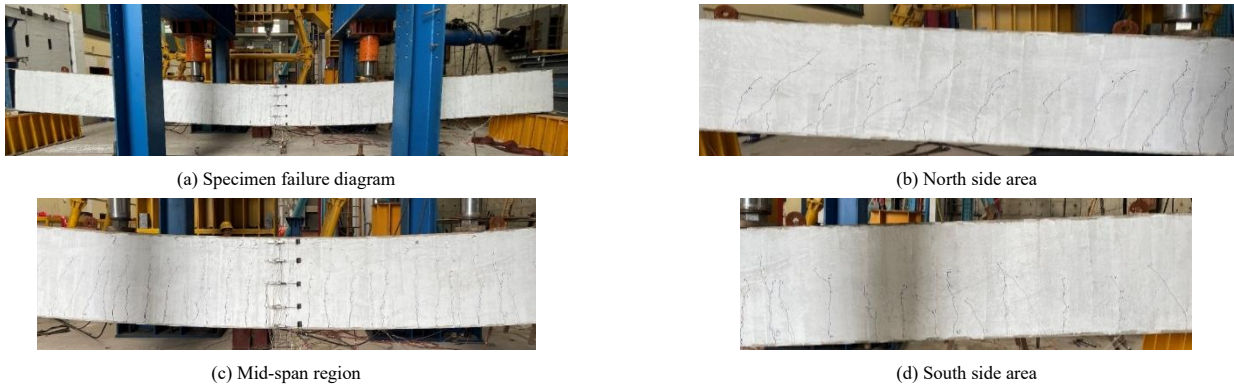
Fig. 4 Final failure state of specimen PECB1
