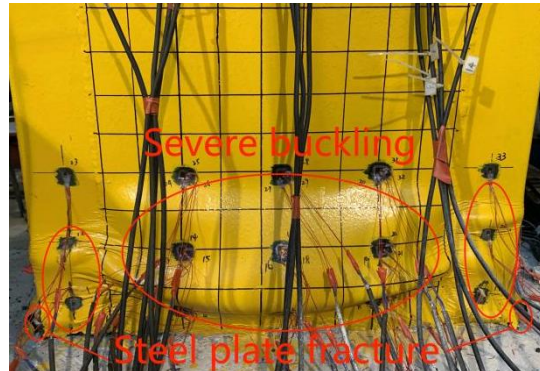
(f) Failure mode of steel plate in SCW-6
