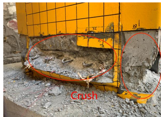
(b) Failure mode of internal concrete in SCW-2
