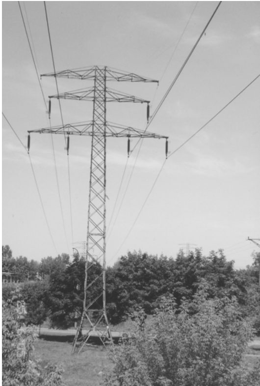
Figure 2. View of Suspension Support
