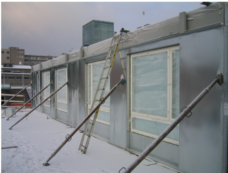
Figure 1. NORDICON Wall Elements with Flat Steel Sheath (As Oy - Arabian Kotiranta; Builder: Sato Rakennuttajat Oy; Architect: Ark Oy Kahri & Co.; Wall: Ruukki)
