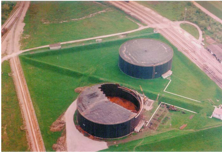
Figure 5. View of Tanks R5 and R6 (R5 during the Rehabilitation Stage)
