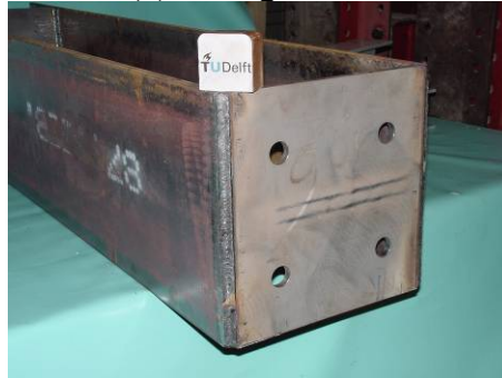
(b) Detail of the Welding of the End Plate to Beam Flange (Outside) for Flush Configuration 2
