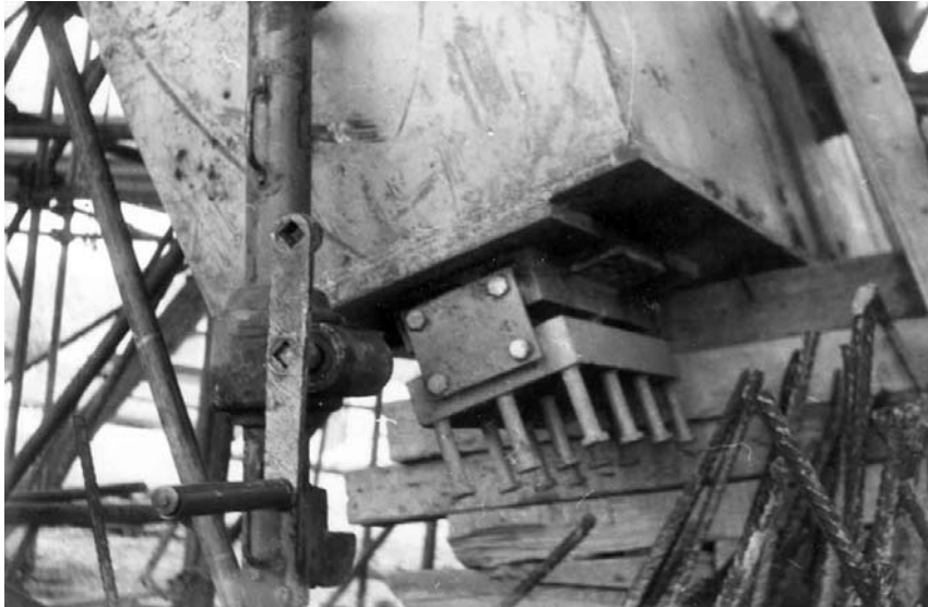
Figure 13. Cylindrical Steel Bearing of the “V”- Supports before Concrete Casting
