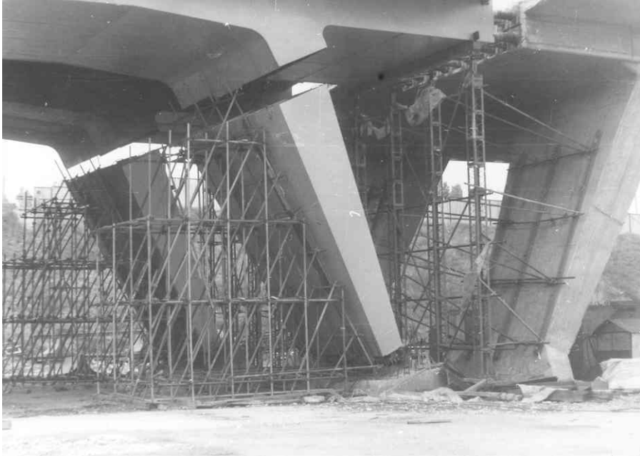
Figure 11. Assembling of the Steel “V”- Supports
