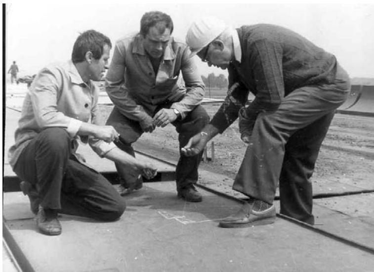
Figure 15. Supervision of the Assembly Process
