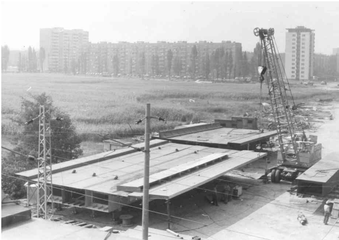
Figure 8. Orthotropic Bridge Storage Yard
