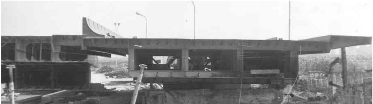
Figure 5. Triple-Box Section of the Bridge Deck
