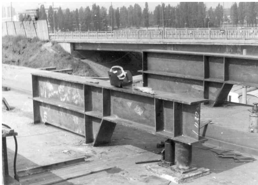
Figure 14. The Fitting Process by Steel Cantilevers and Hydraulic Jacks
