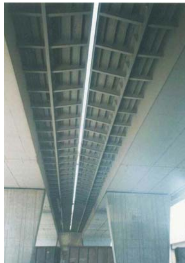
Figure 18. A View from Beneath the Orthotropic Bridge
