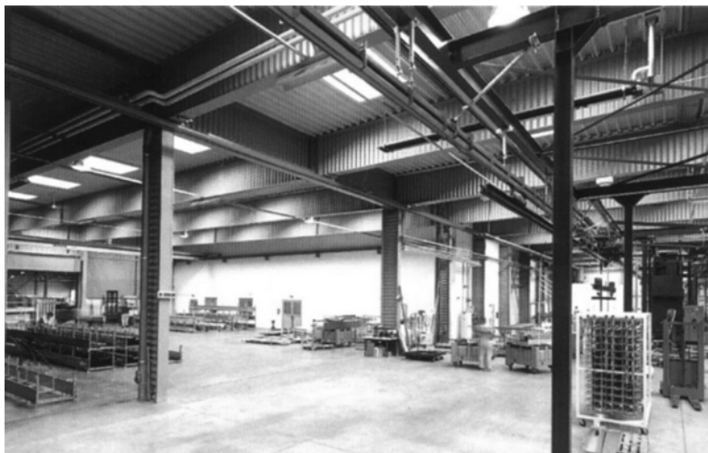
Figure 3 Industrial Hall Made of Girders with Corrugated Web
