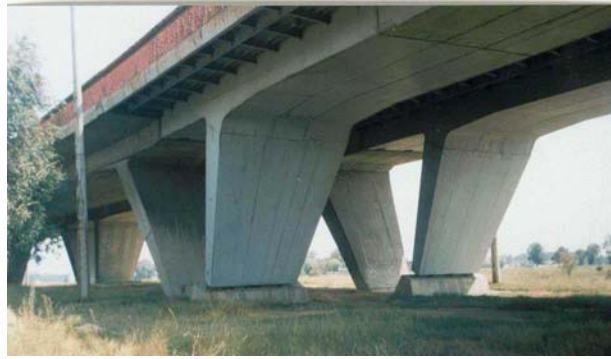
Figure 17. A View of the Steel and Concrete Parts of the Bridge
