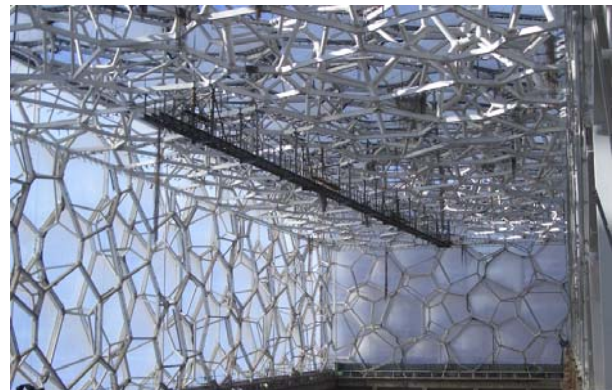
Figure 2. Interior view of Water Cube (in construction)
