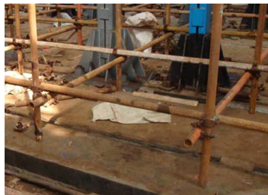
Figure 5. Bottom of the Falsework System
