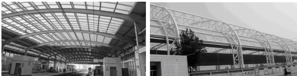
(a) Xianglujiao Light-rail Station
