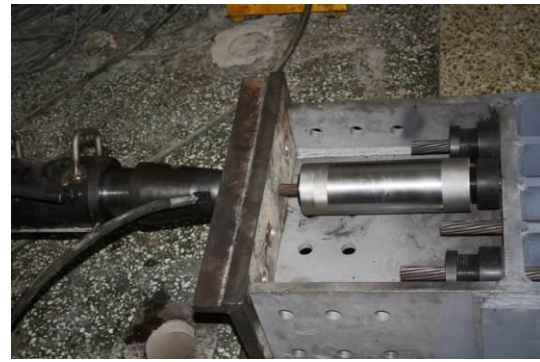
(b) Connecting transformation casing and pre-tightening of the tensioning anchor
