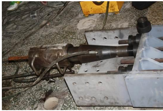
(a) Pre-tightening of the anchorage end
