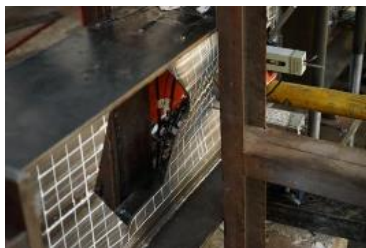
(a) Local buckling of the webs between the holes in the loading process
