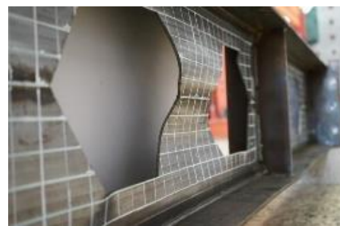
(b) Local buckling of the webs
