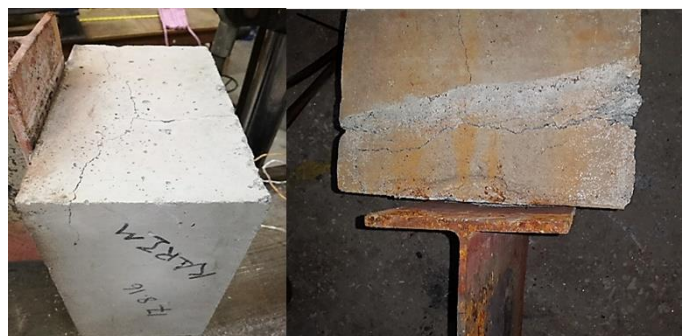
Fig. 12 Cracks on concrete slab after connector specimen failure at elevated temperature
