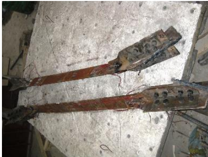
(b) Buckling of inner core of BRBs after disassemble
