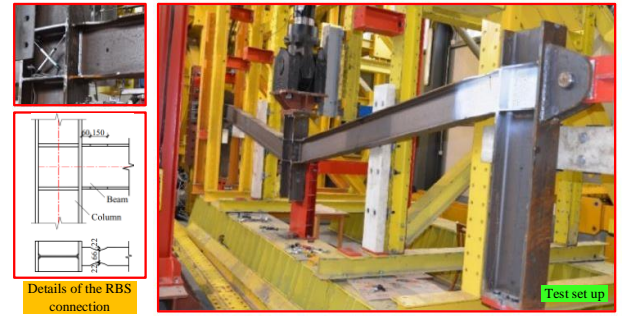
Fig. 4 Collapse test of one-story steel frame with RBS connection [6] (dimension units: mm)
