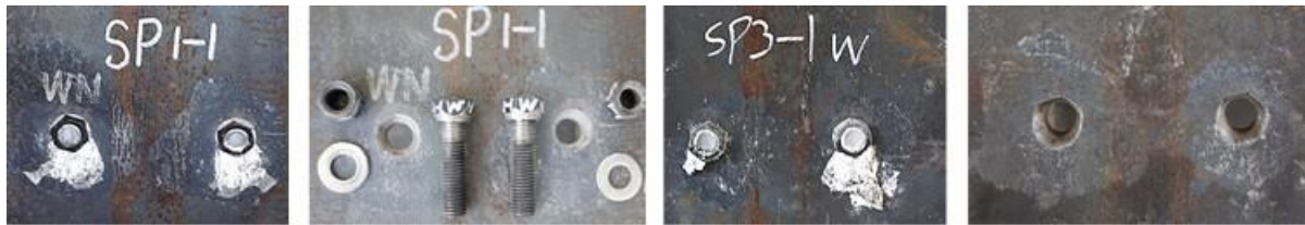
(c) Steel beam flange after removing failure bolts
