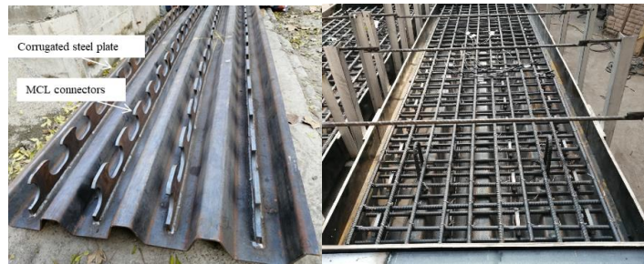
(a) Fabrication of the steel structure (b) Erection of the formwork
