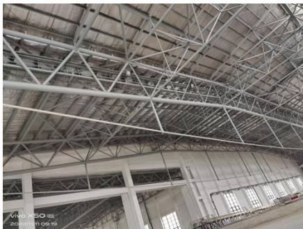
(b) Tension beam structure
