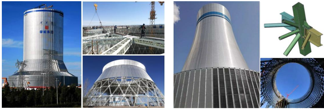
(a) The 181 m high cooling tower with welded joints
