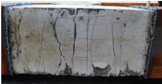
(a) Tensile side of sandwich concrete
