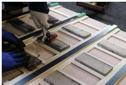
b) Removing by a scraper
