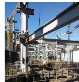
(c) Construction of weather-resistant steel frame
