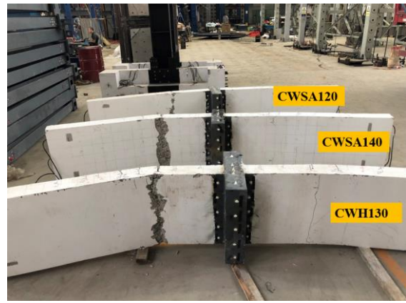
(b) Deformation and concrete fracture
