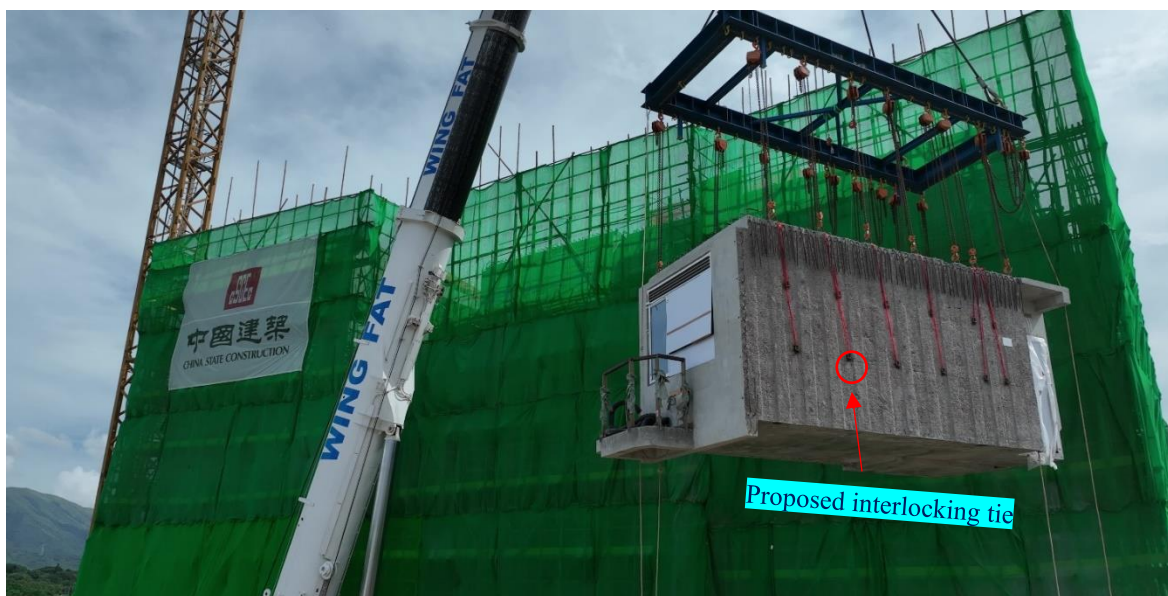
Fig. 29 Proposed interlocking ties adopted in a MiC building
