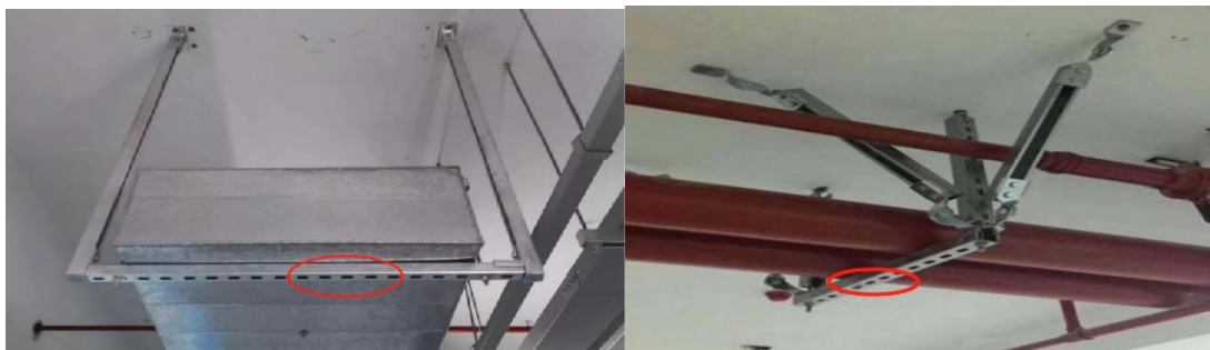
Fig. 1 CFTWS in prefabricated support and hanger
