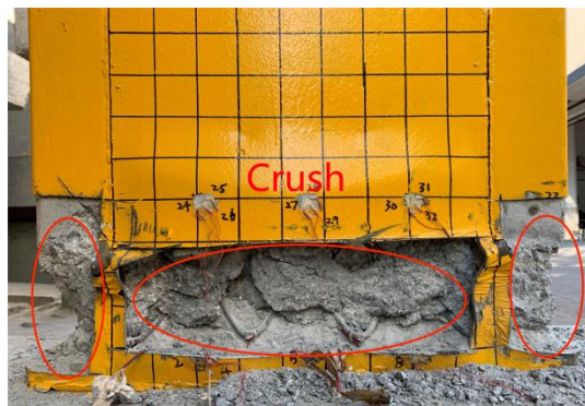
(c) Failure mode of internal concrete in SCW-3
